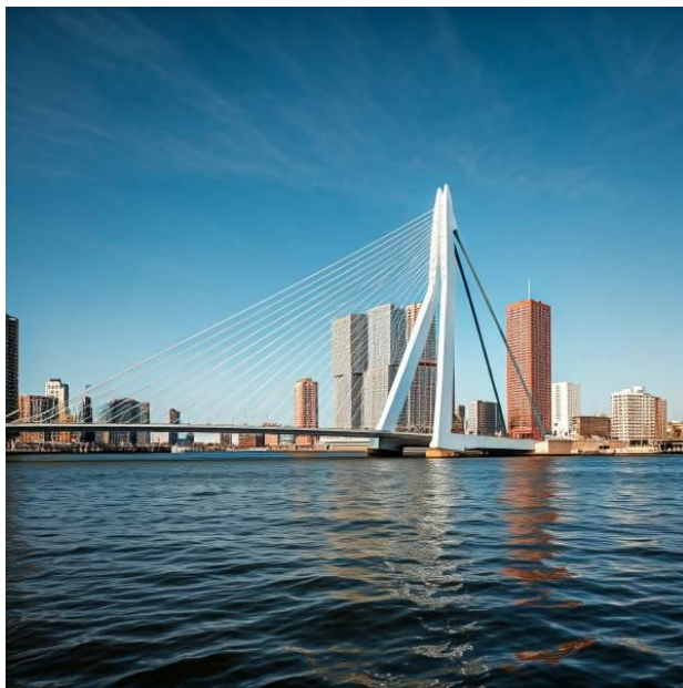
Erasmus Bridge in Rotterdam, Netherlands:
